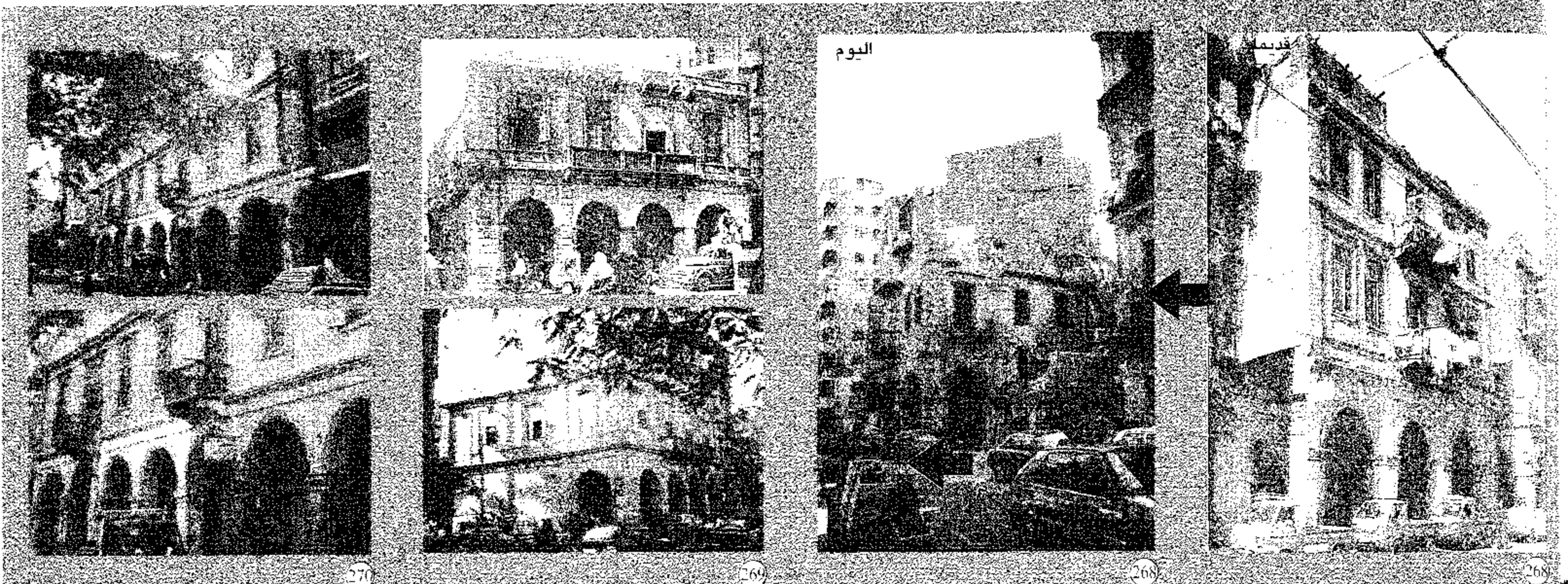
72 & 74 El-Qalaa St. Built : about 1880 No. of storeys : unknown today only 2 left Style : Classic - among bldgs. with pedestrian arcades
